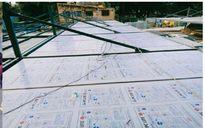
Honeycomb Sheets for Parking Shelter, Bosch, Bangalore
