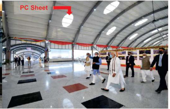
PC Profile Sheets Supply for Railway Station, Bhopal
